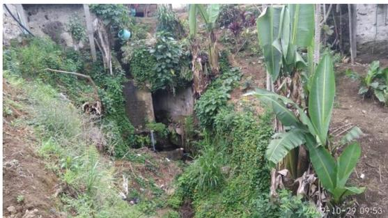
**Figura 174. Box Culvert- taludes inestables**
